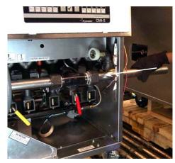
Figure 3. Insert drainpipe section into fryer drain-tee before pushing fryers together (arrow). Do this as required for all cabinets being assembled.
